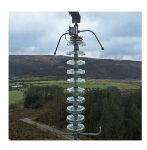
We produce glass insulators, the "disk-shaped" insulating parts used on high-voltage lines, at our Spanish site. As part of our efforts to help our customers reduce CO<sub>2</sub> emissions and the additional costs associated with overly frequent cleaning or electrical bypasses caused by a lack of maintenance,
